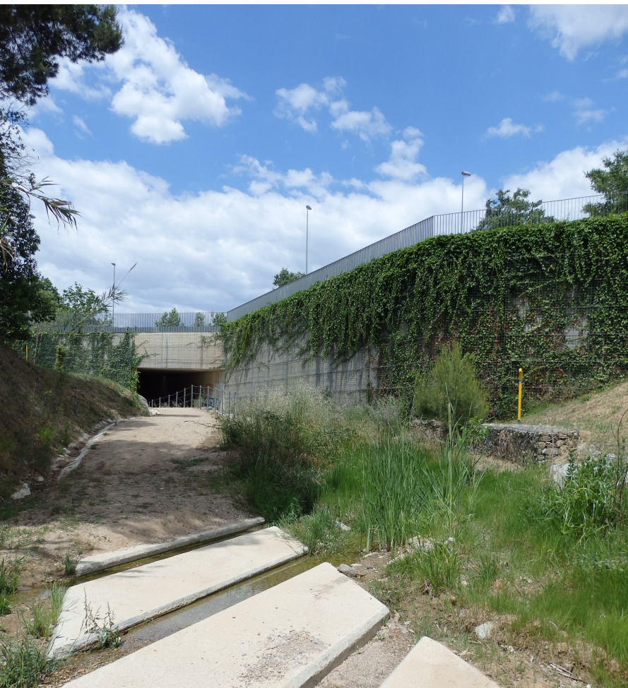
Torrent de Sant Marçal and its passage under the BP-1413. In the foreground, ford over the riverbed for amphibians.
