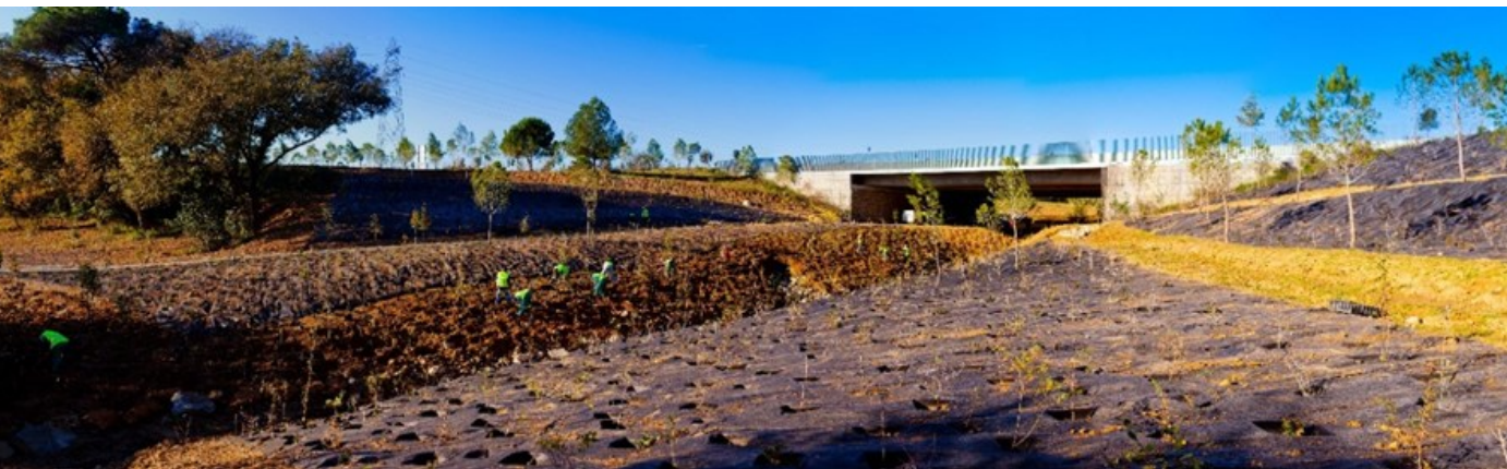
Planting works in the green corridor in the riverbed of Torrent del Bosc
