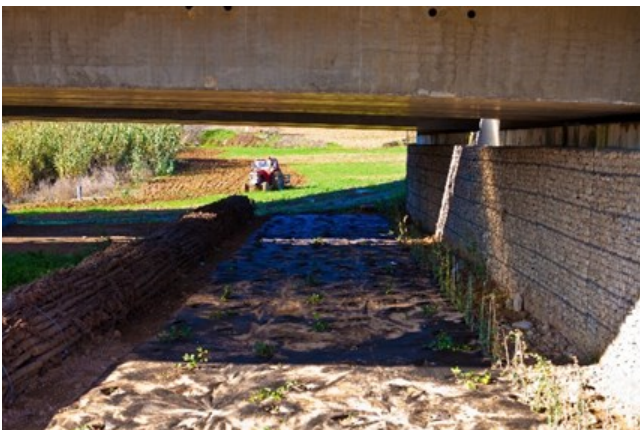
Close-ups of the adaptations made to the Torrent de Can Fatjó viaduct to favour the crossing of fauna, which integrate sanctuaries for small fauna like insects, invertebrates and micromammals.
